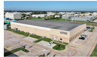
Houston, TX 50,000 square foot fabrication facility Metalforms Heat Transfer
